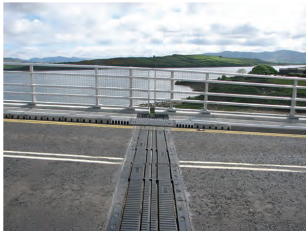
Bridge expansion joints, like this one on the Harry Blaney Bridge in County Donegal, Ireland, allow for expansion and contraction of the asphalt and steel without damage to the bridge. (Image credit: Willie Duffin)
